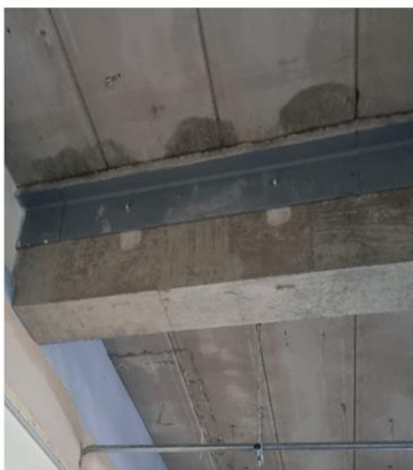
End bearing strengthening
